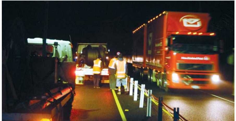
Workers installing wire rope barrier on Centennial Highway.
