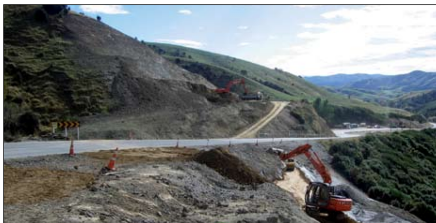
Work is underway on the Tunnel Hill realignment project.
