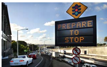
Electronic sign 'Prepare to Stop' advises motorists of ramp signals ahead.
