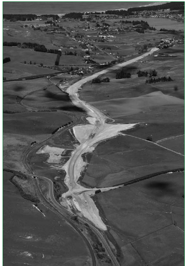
An aerial view of the Tumaï realignment project.
