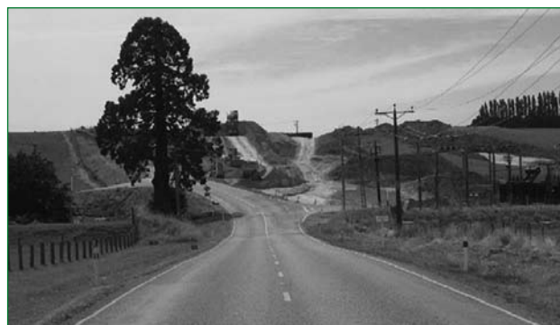
The realignment work on River Road, SH93.
