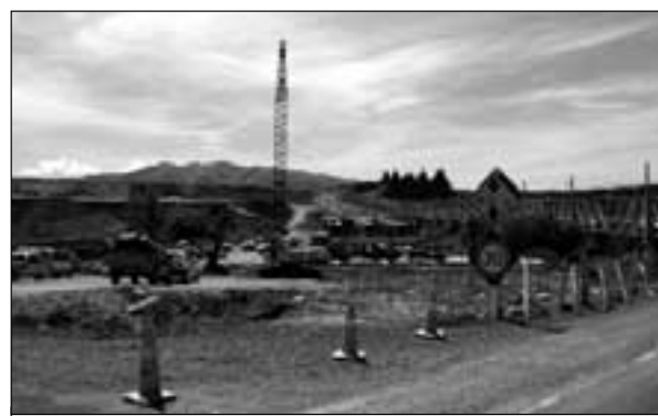
The view north looking at the Awatere River bridge construction.
