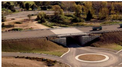
The new roundabout at MacKays Crossing, also constructed as part of the project, with the old road in the background.
