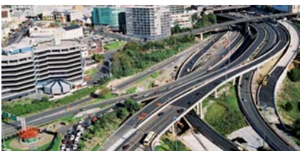
Aerial view of Central Motorway Junction as the project nears completion.
