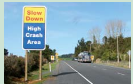
SH27 large warning signs alert motorists to the crash risk
