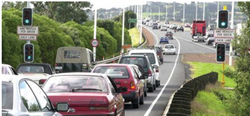
SH20 Southwestern Motorway on-ramp at Rimu Road where ramp signals have undergone an earlier trial.
