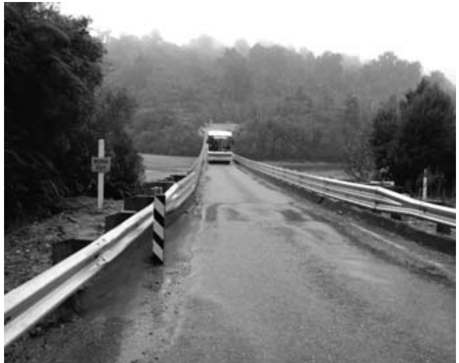
Steel guardrails have replaced wooden handrails at Waitaha Bridge on SH 6.
